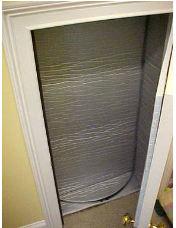
Attic Tent Vertically installed
